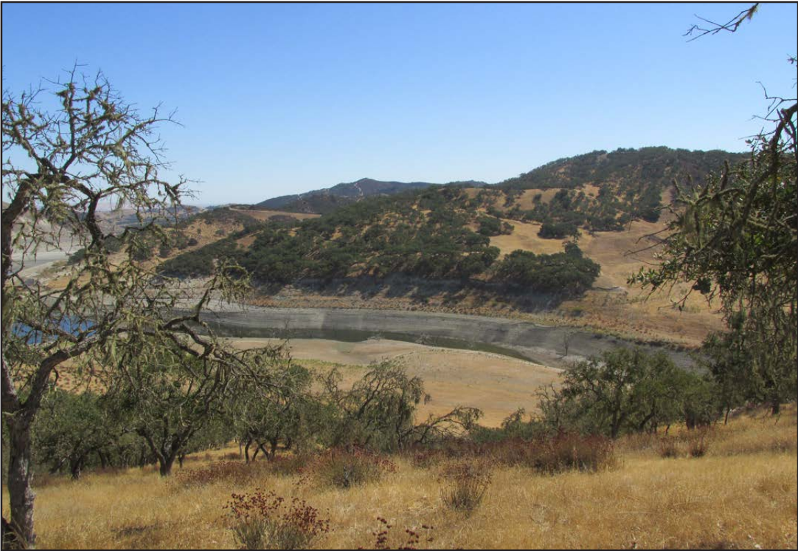
Key View 7. Looking east-southeast from a dirt road north of Interlake Road toward the Energy Dissipation Structure work area at San Antonio Reservoir.
